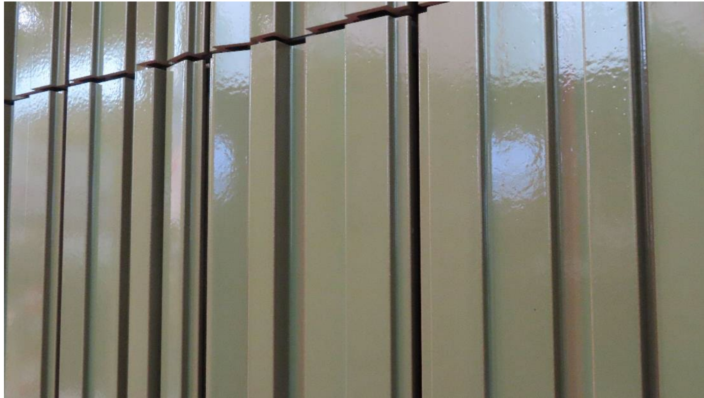
TONALITY® - mounted with V-UK / system with open vertical joint (at least 10mm) - all UK components are painted black
